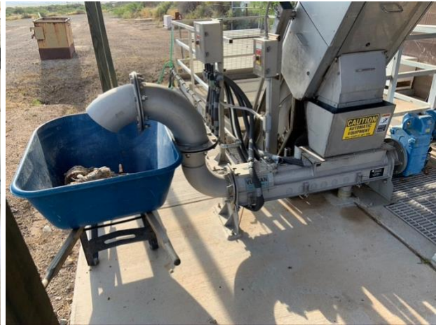
Barscreen with washer/compactor (Lordsburg WWTF)
