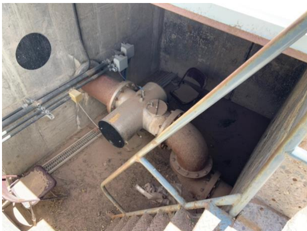
Photo #6 UV Disinfection Unit
