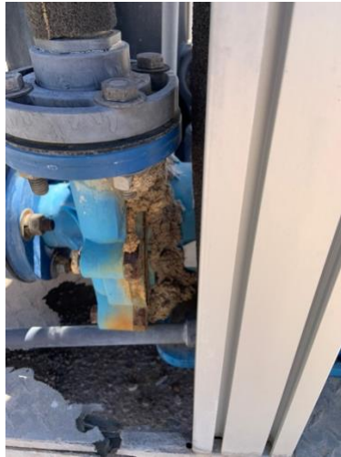
Photo #2 Hydroxide Pump
