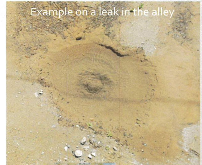
Example of a leak on Veater
